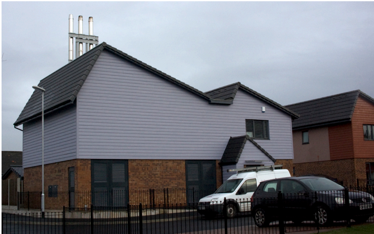
Figure 1 The energy centre at the Park Dale zero carbon housing development in Airedale, West Yorkshire (note the asymmetrical roof and the three chimneys for the biomass boiler)
